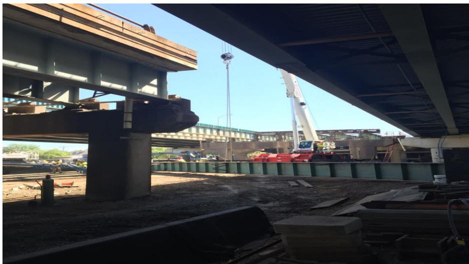
Removal of Br. 163 Span 10 Steel Girders
