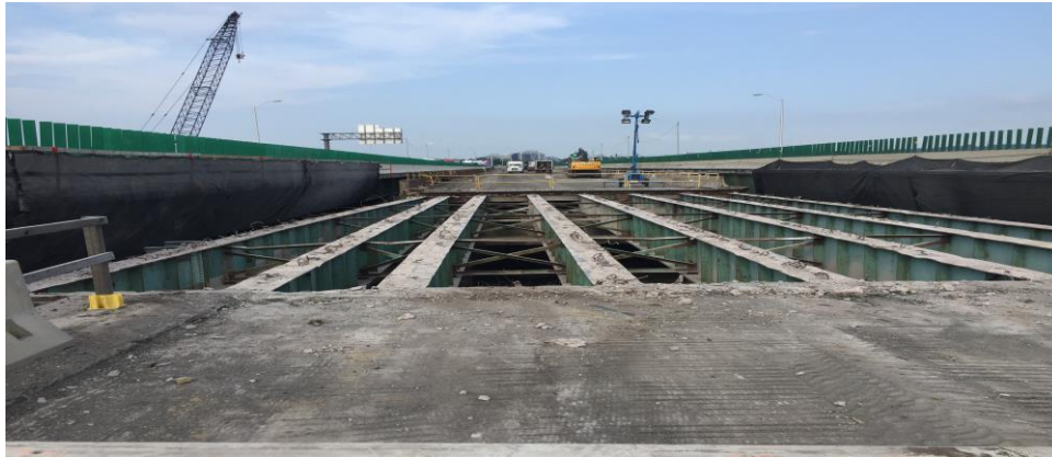
Removal of Br. 163 Span 10 Deck
