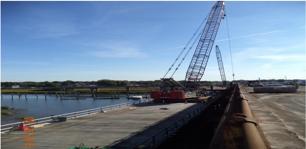
Existing Bridge No. 163, Asphalt Removal prior to Demolition
