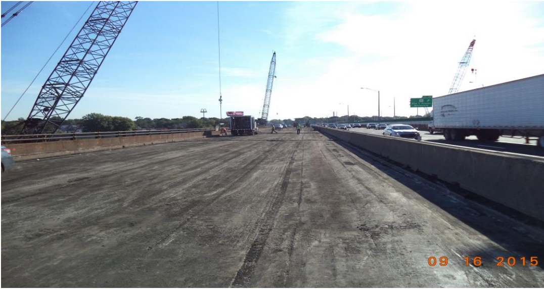
Existing Br. No. 163 & Stage 2 Temporary Work Trestle
