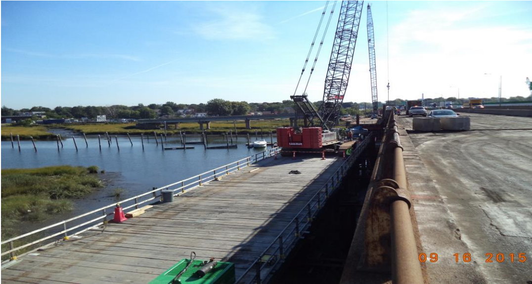
Existing Bridge No. 163 & Stage 2 Temporary Work Trestle
