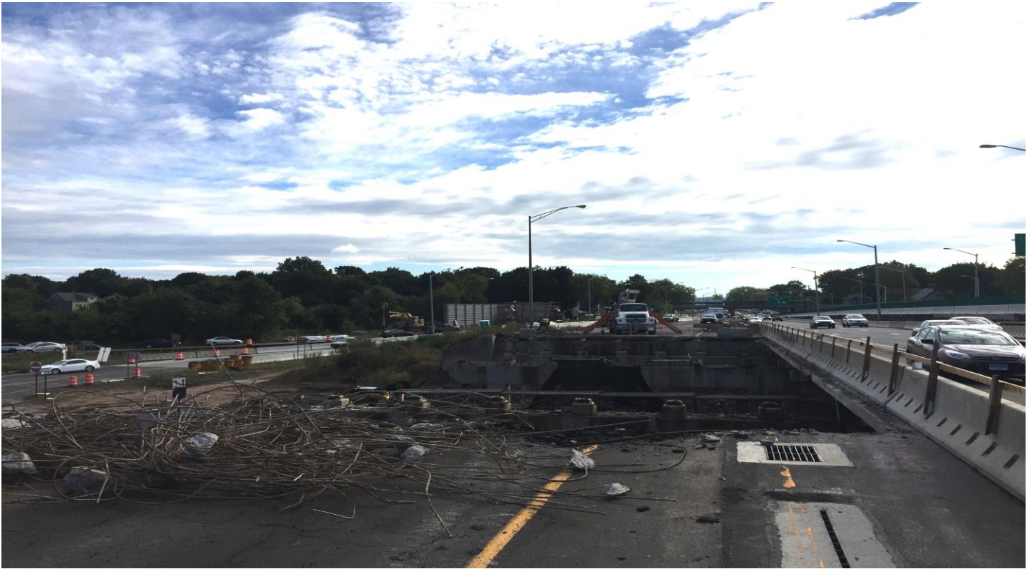
“Full Size Render” : Bridge No. 164 Stage 2 Demolition
