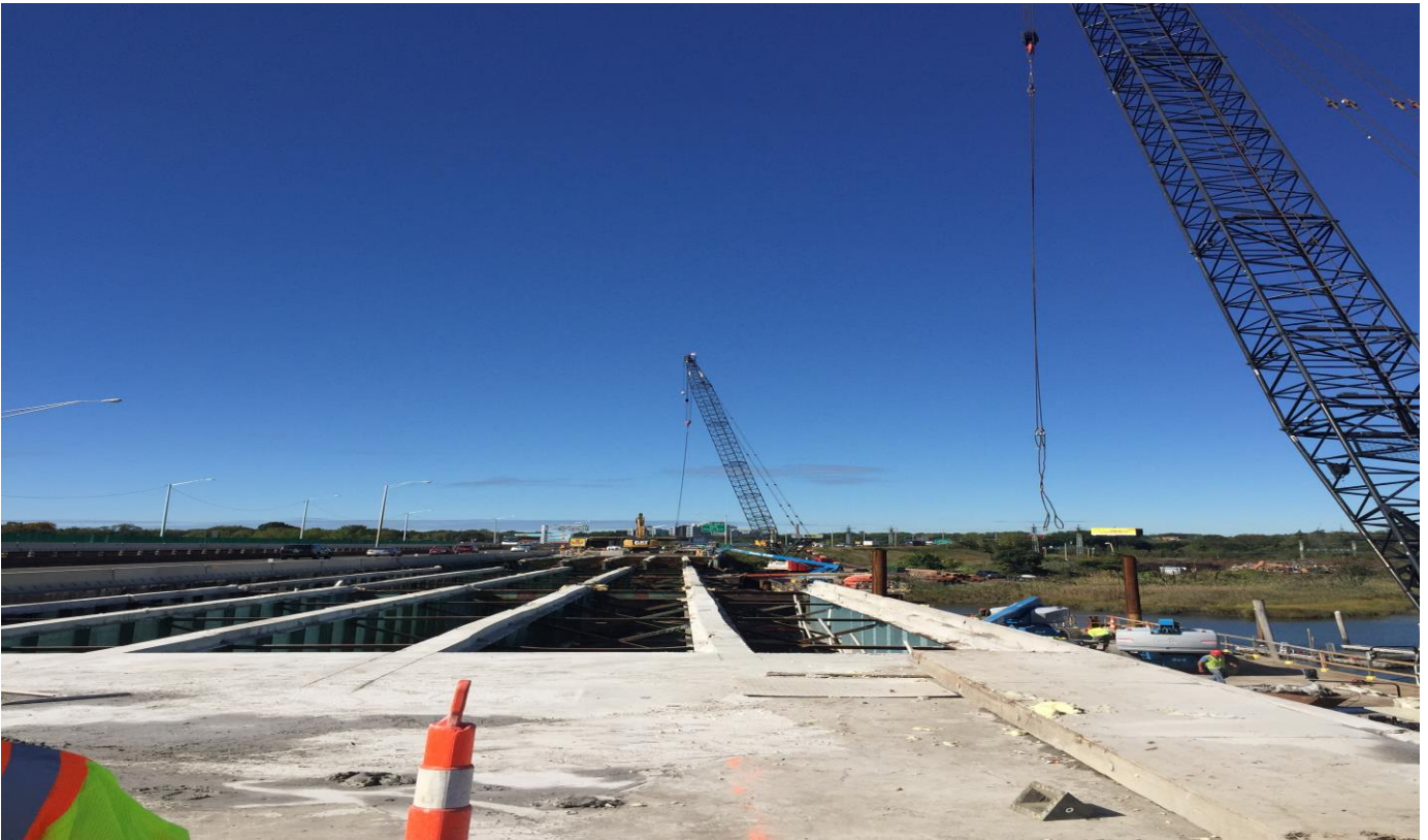
“Deck Removal of Bridge 163”
