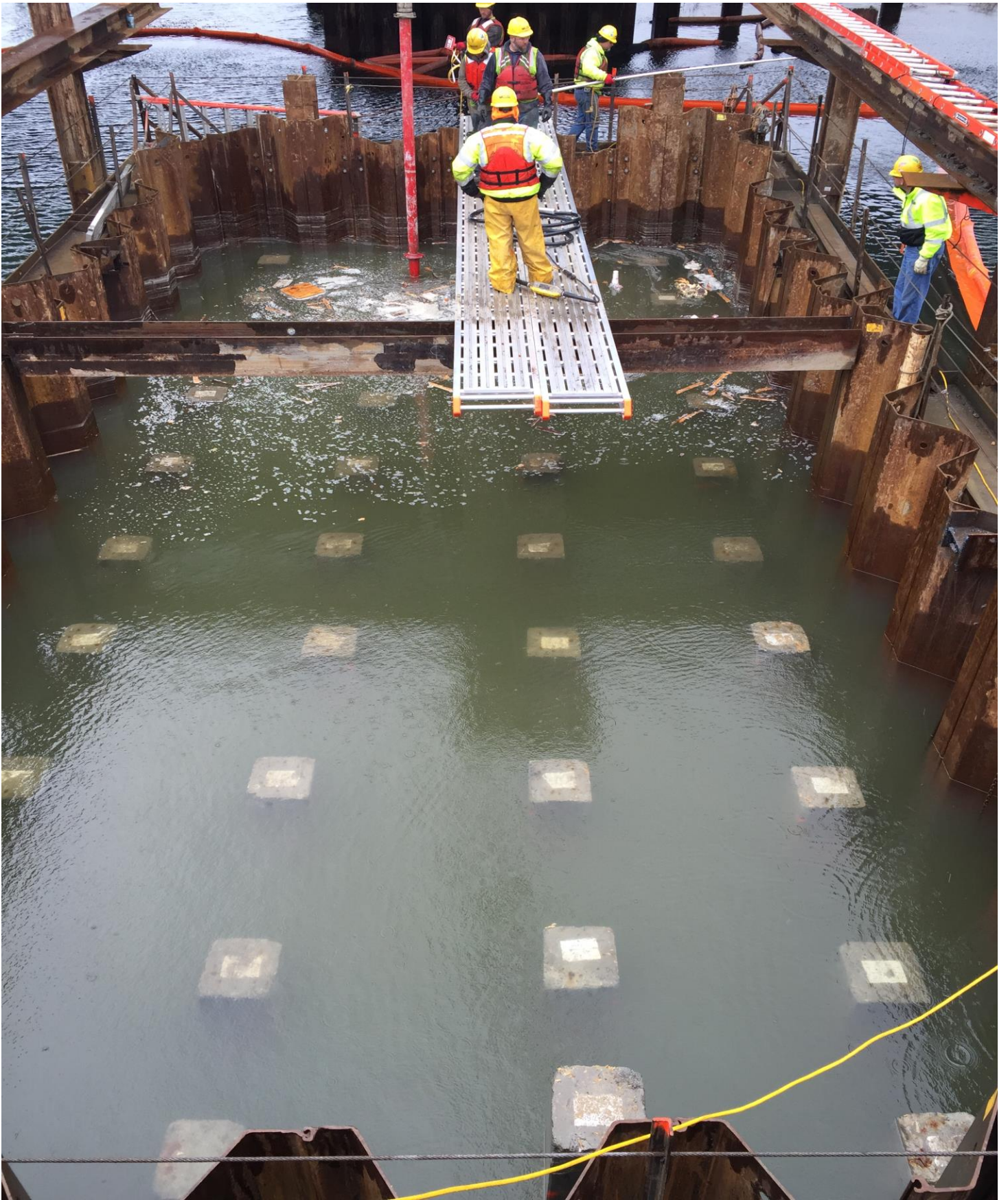
“Bridge 163 Stage 2, Pier 2 Driven Piles
