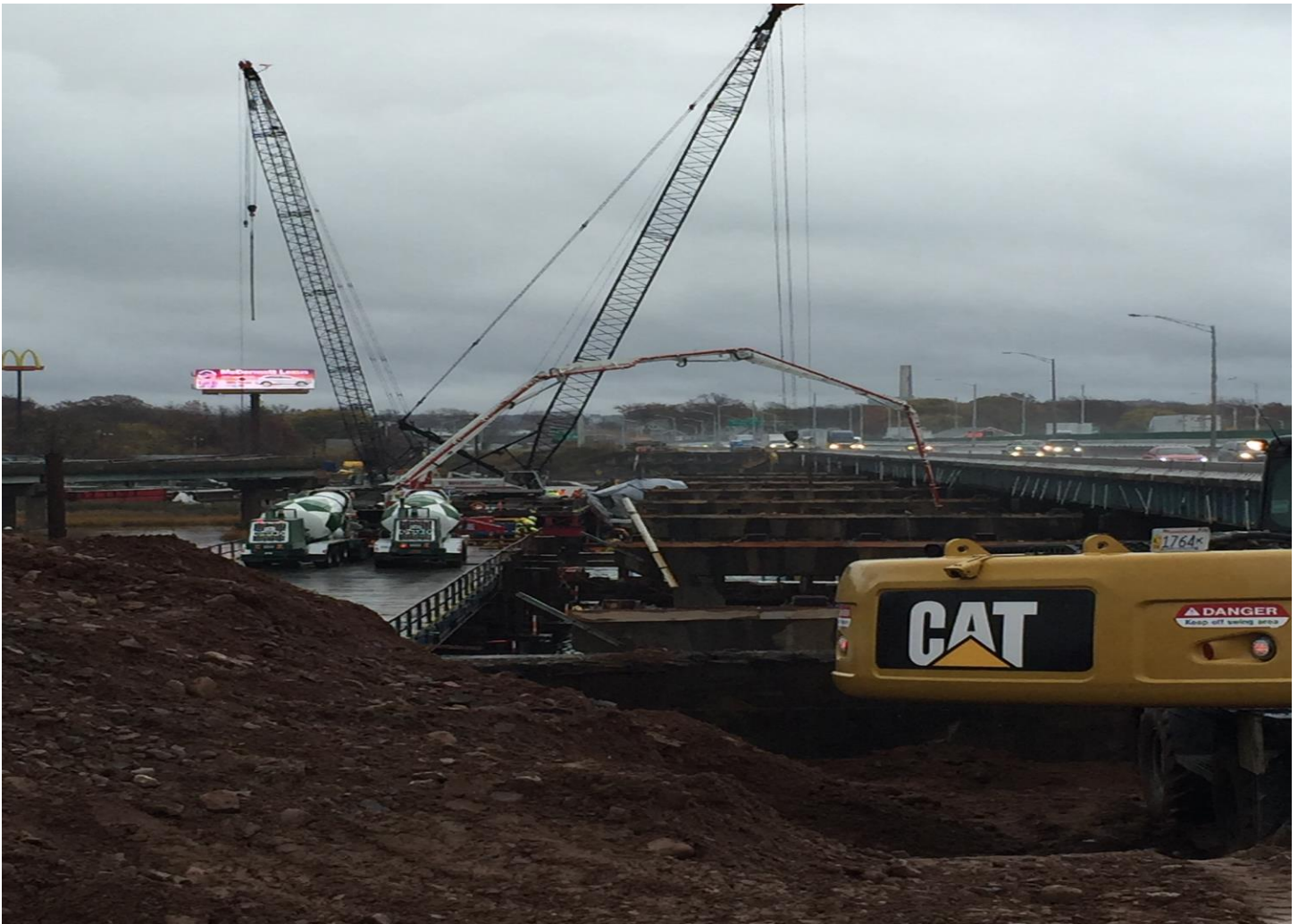
“Bridge 163 Pier 2 Tremie Concrete Pour”
