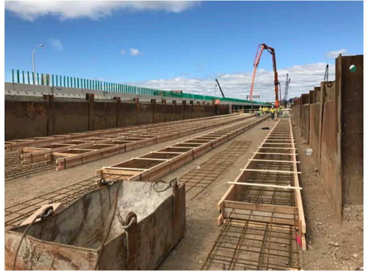
Footings for Steel Launching
