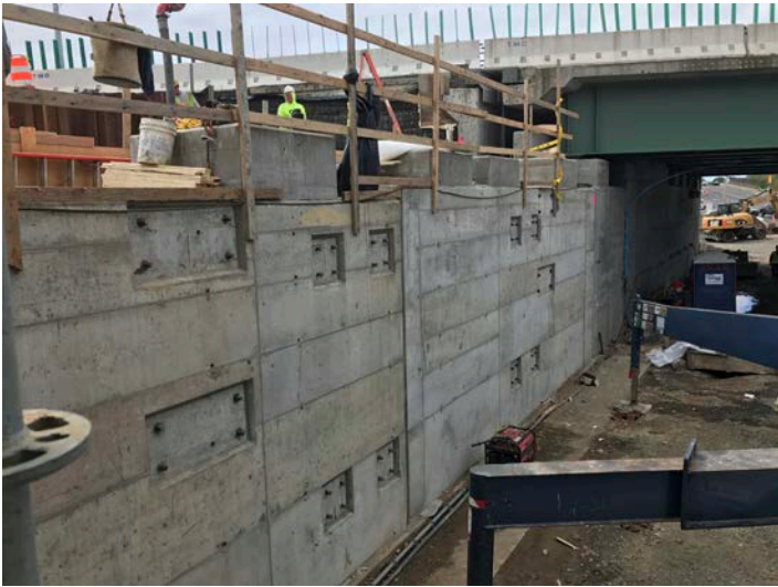
Bridge No. 163 Abutment 2
