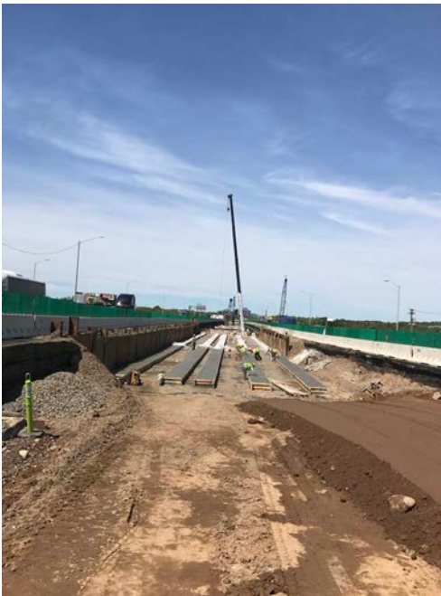
Footings for Steel Launching
