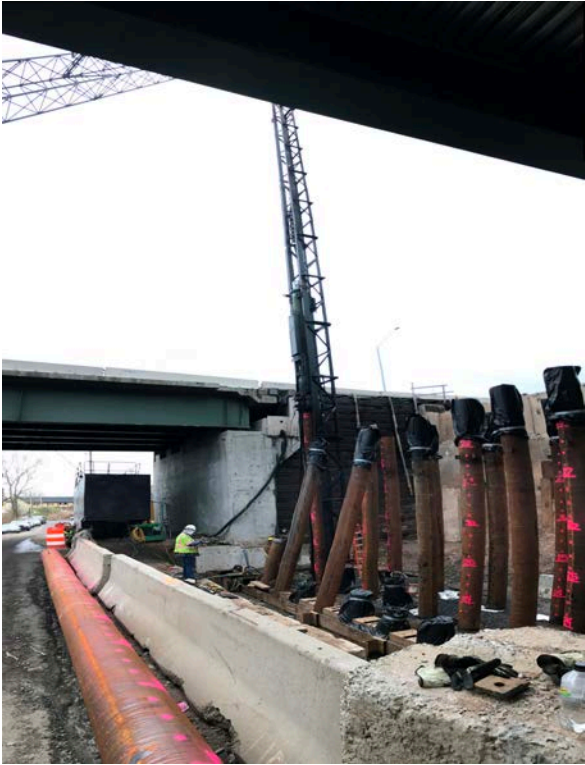
Driving Tapertube Piles at Br. 163 Abutment 1
