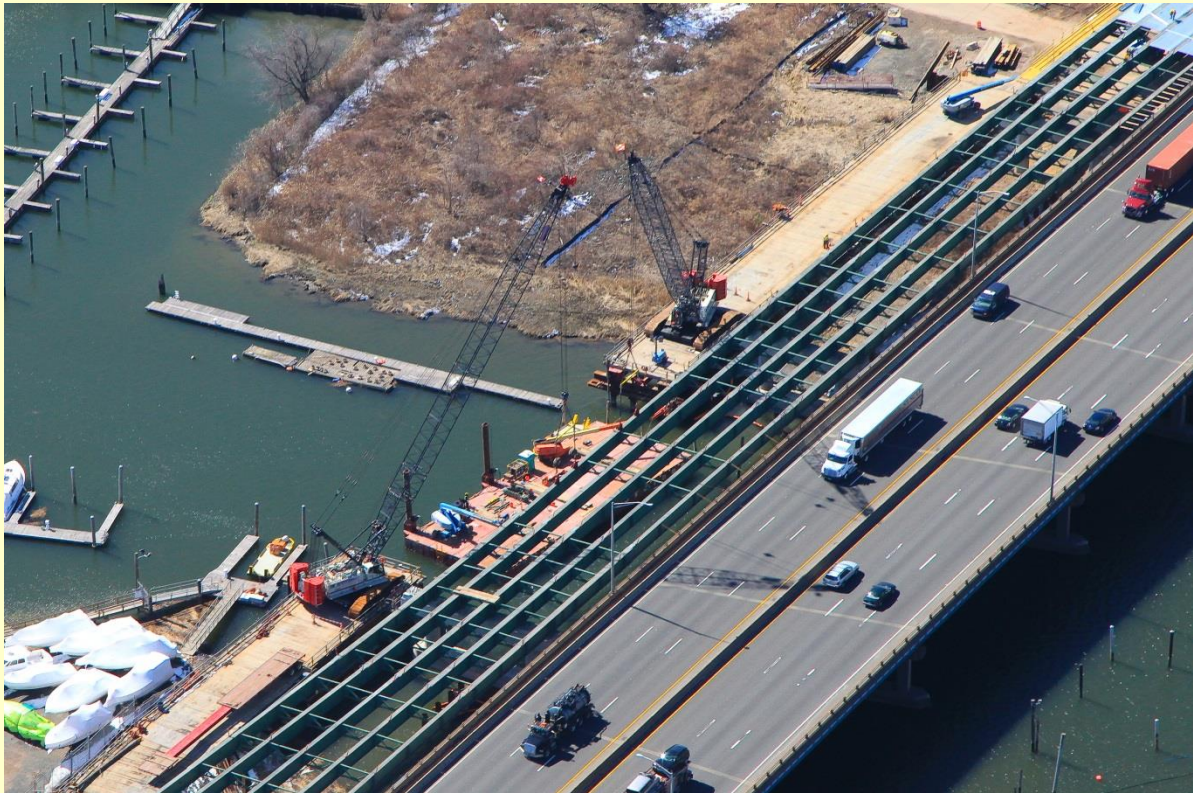
Bridge 163, Stage 1 Structural Steel Erection
