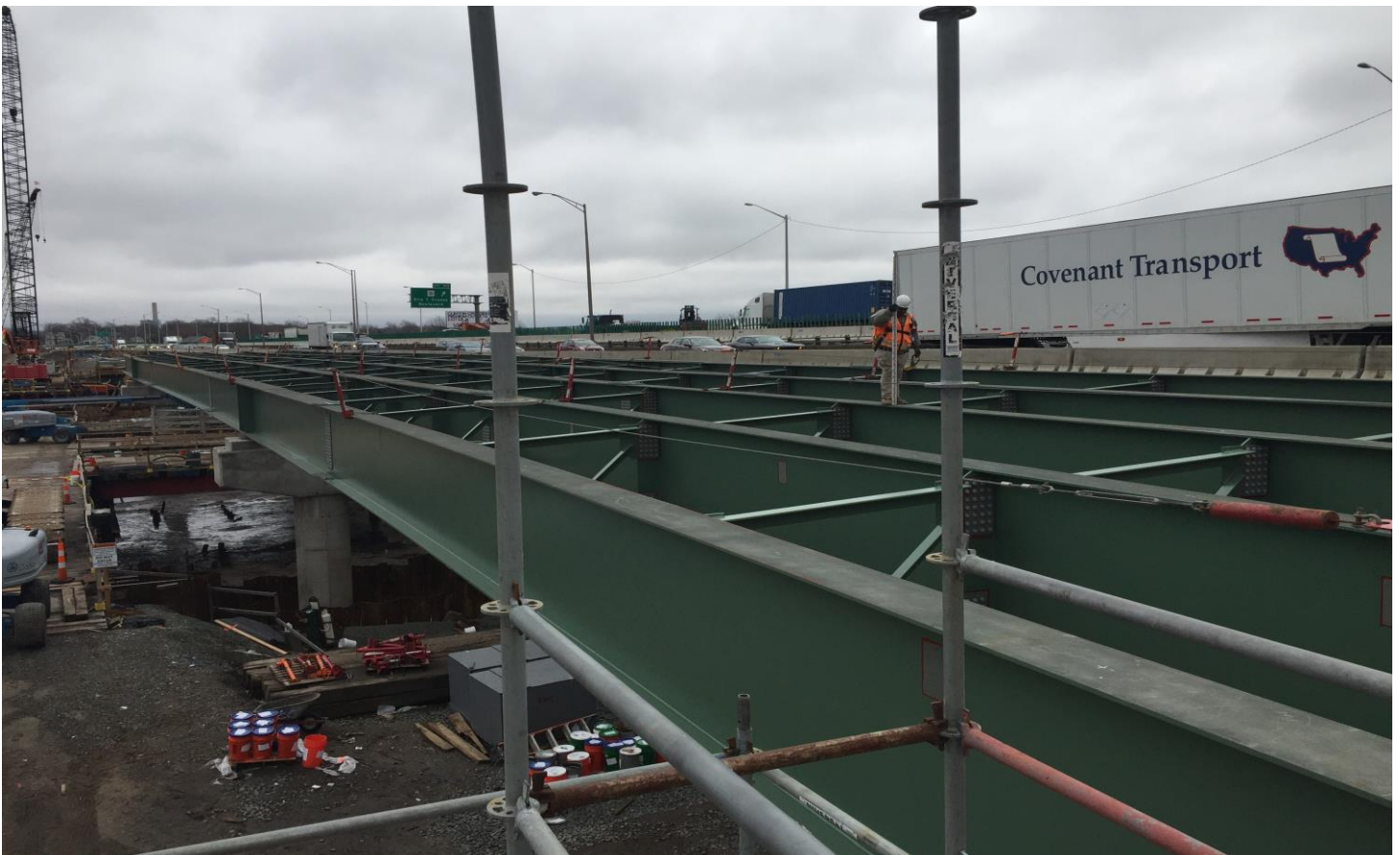
New Bridge 163 Structural Steel, Looking East
