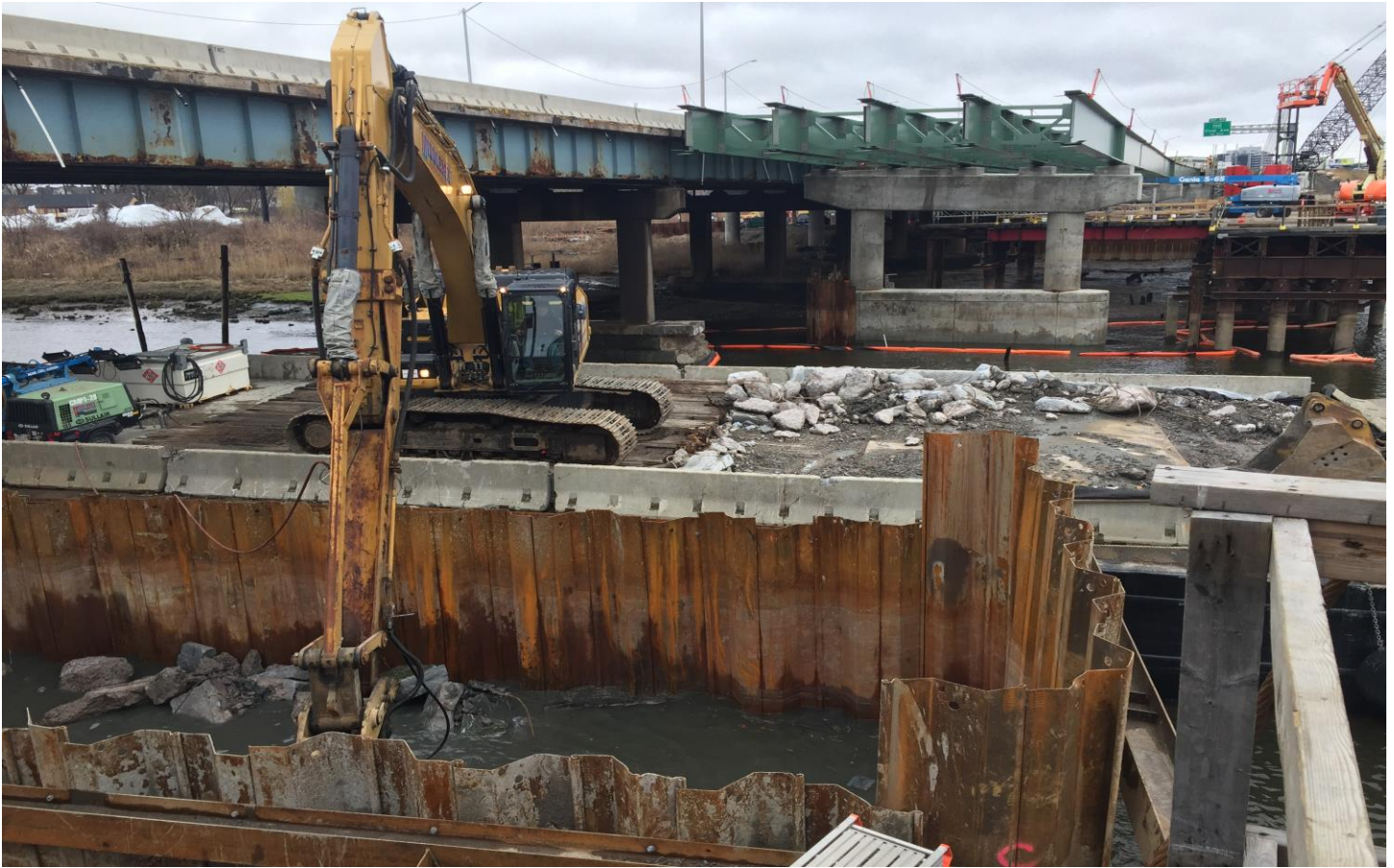
Demolition of Existing Bridge Pier
