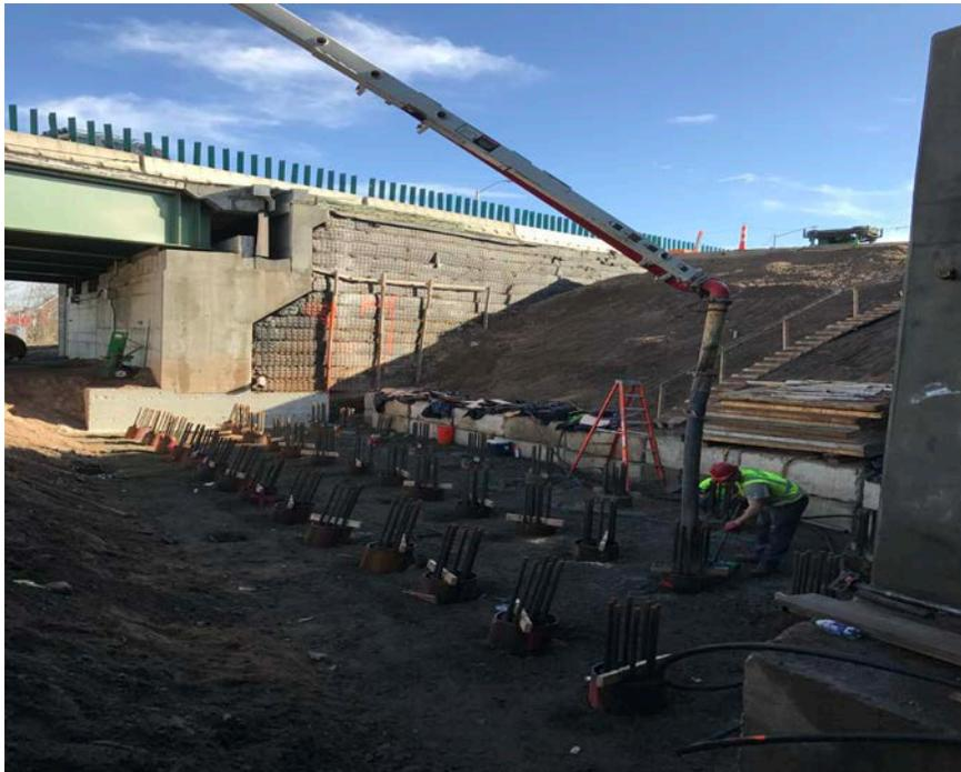
BR163 Abutment 2 Stage 3 Piles Being Grouted
