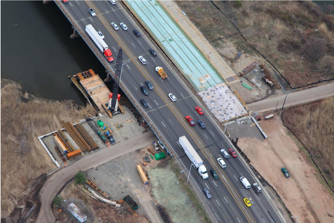
Bridge 163 West approach
