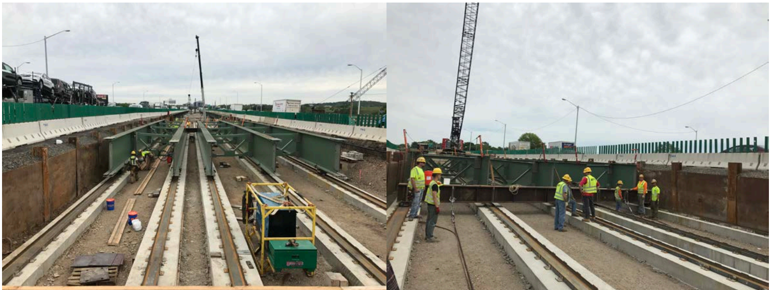
STEEL LAUNCHING OPERATION
