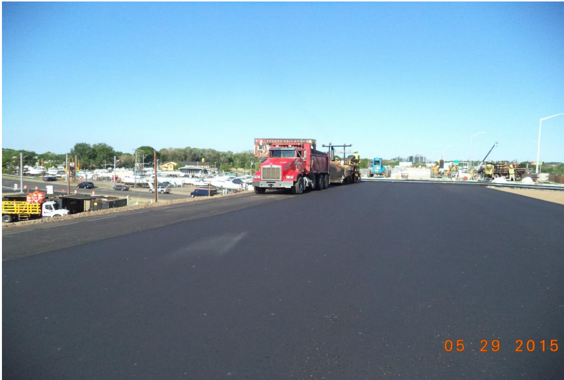
New Pavement – I-95 NB Exit 44 off ramp
