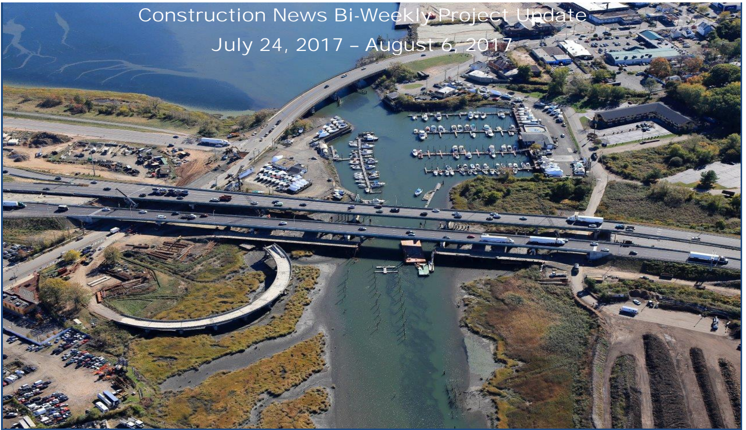
Rehabilitation of Bridge No. 00163A, I-95 over West River and State Route 745 in the Towns of West Haven and New Haven
