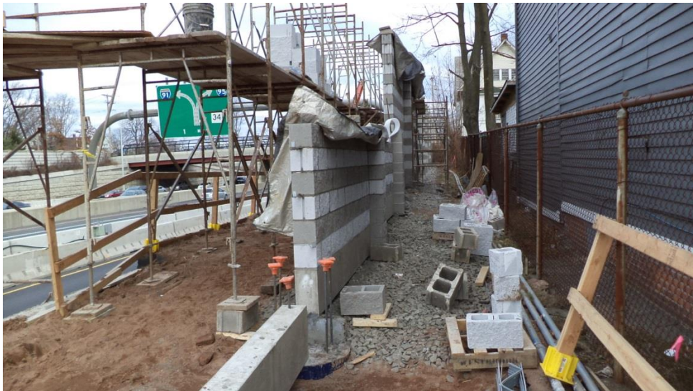
New noise barrier wall along of I-95 NB
