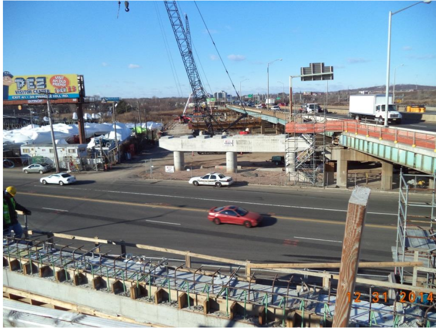
Building of new Pier 5
