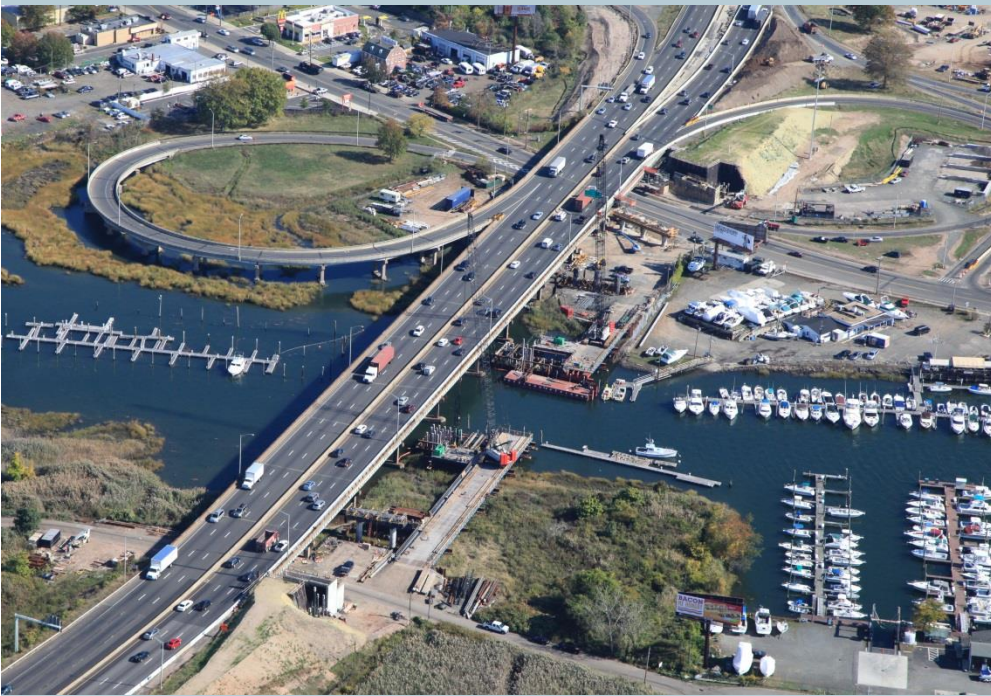
ARIAL VIEW OF I-95 NB &amp; SB OVER WEST RIVER BRIDGE
