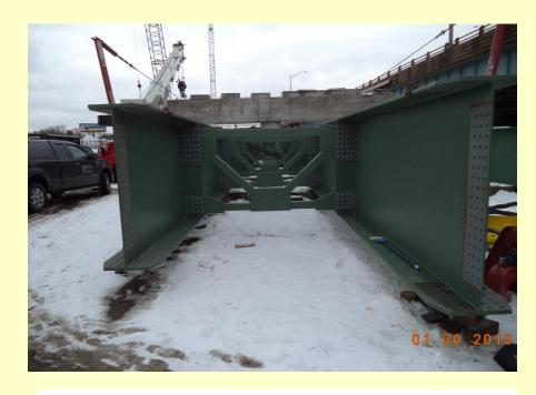
Bridge 163 structured steel assembled on the ground
