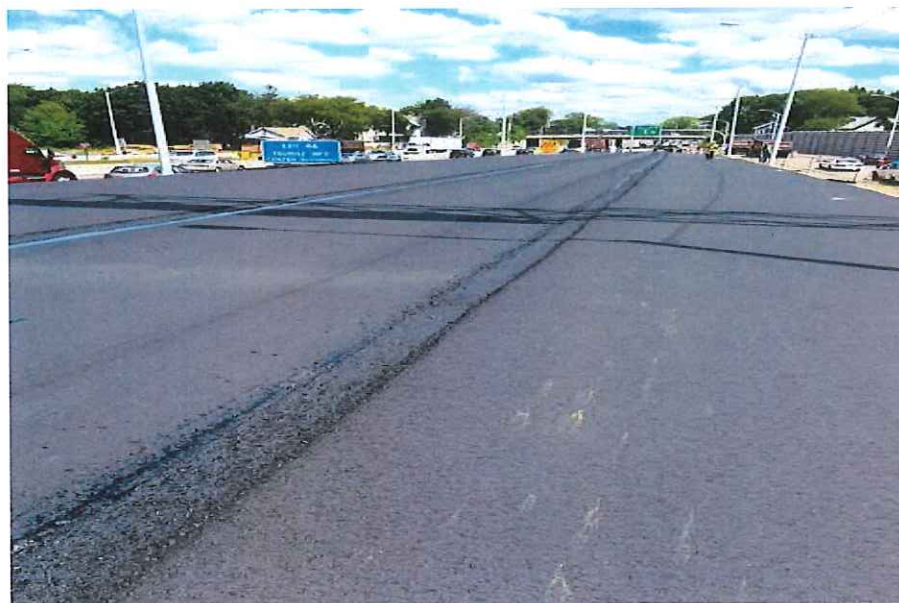
PAVING I-95 NORTHBOUND-NEW BRIDGE-OVER THE WEST RIVER
