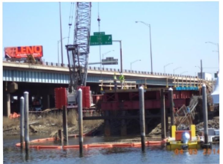
East trestle, South of I-95 NB
