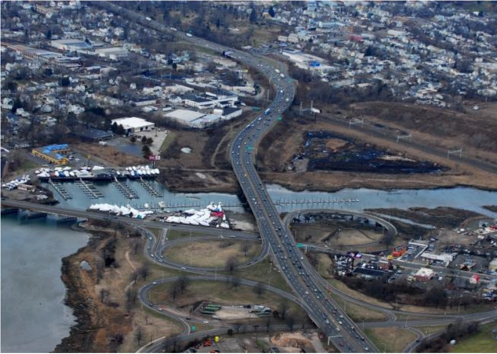
ARIAL VIEW OF I-95 NB & SB OVER WEST RIVER BRIDGE
