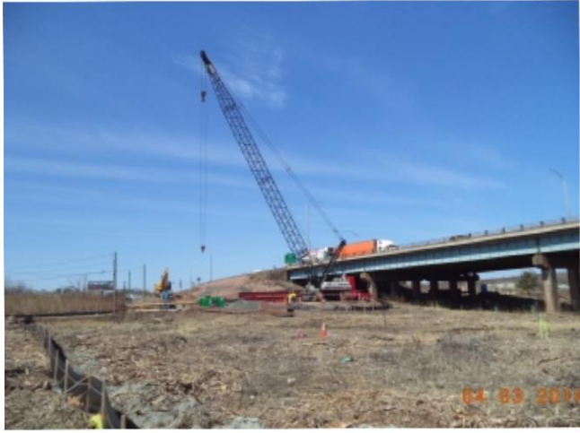
West trestle, South of I-95 NB
