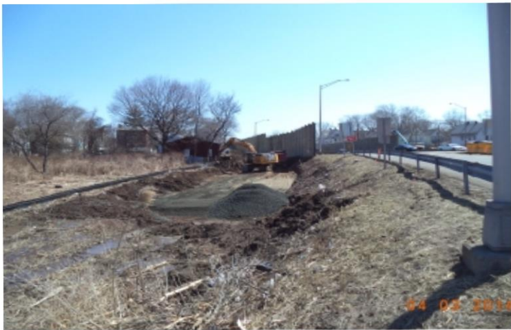
Excavation of material, PLA-2 North off Exit 45 SB off ramp
